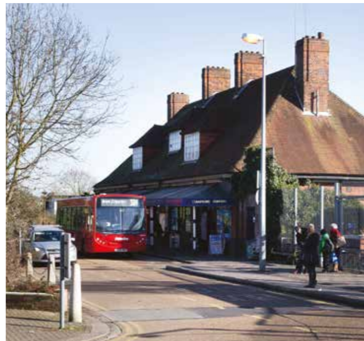
Stanmore Station forecourt
