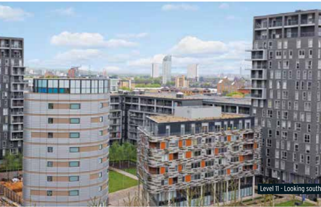
Level 11 - Looking east
