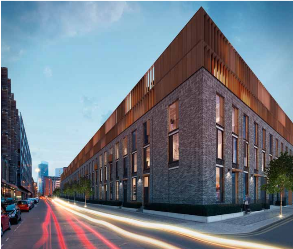
The pioneering Roof Gardens, One Ellesmere Street
